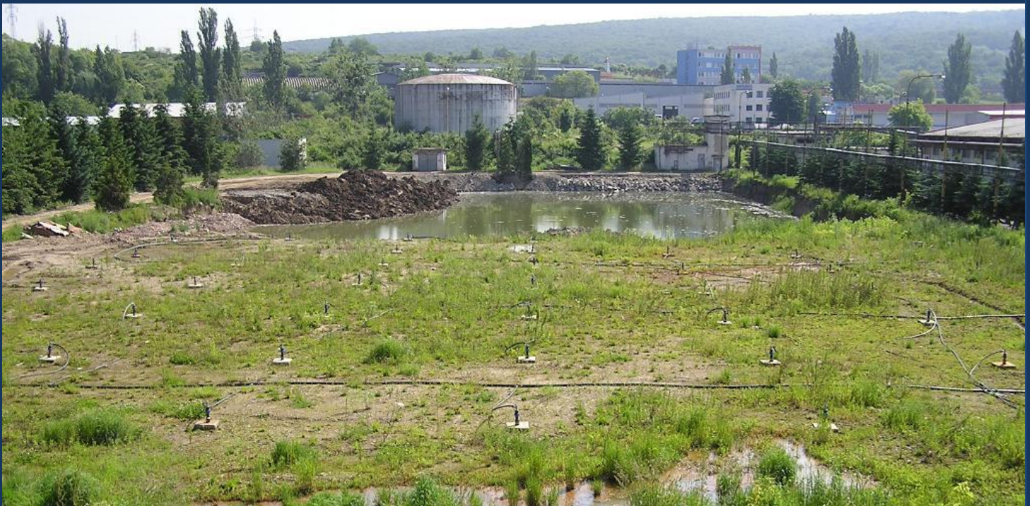
Slovakia - Former fuel storage site remediation, Photo J.Džupír
